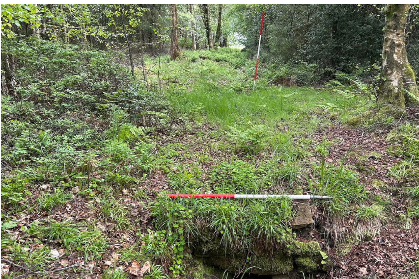
Figure 18. View looking south of culvert in Feature 12 ditch at 12a crossed by track Feature 17 from left to right on the photograph.
