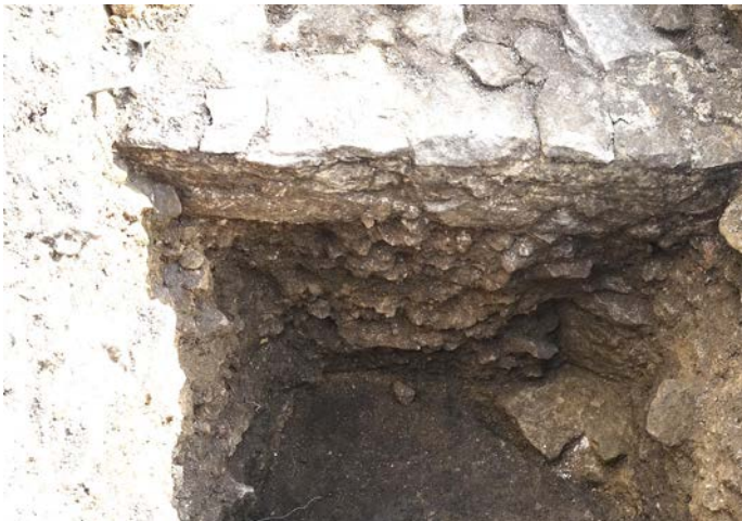
Figure 7. View looking south of Sondage A showing the wall of Building 1 (F9031) in the right hand corner of the trench cutting the dark organic soil 9042. Note the raft of stone rubble below the coursed stonework of the plinth (F9026).
