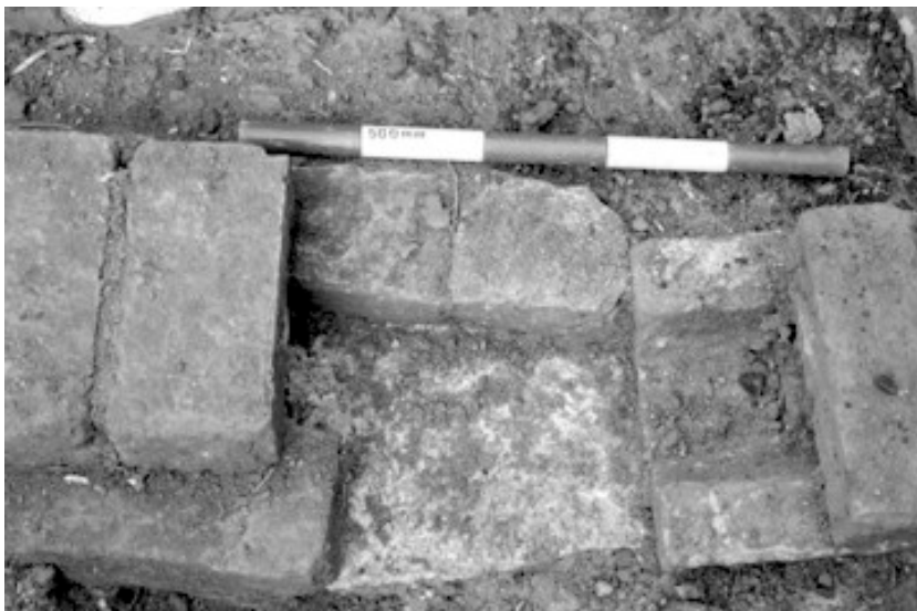
Figure 13 (above): Exposed inlet channel following the removal of some of the capping bricks – carved stone channel on the right, closest to the well house; flat stone 'floor' to the left
