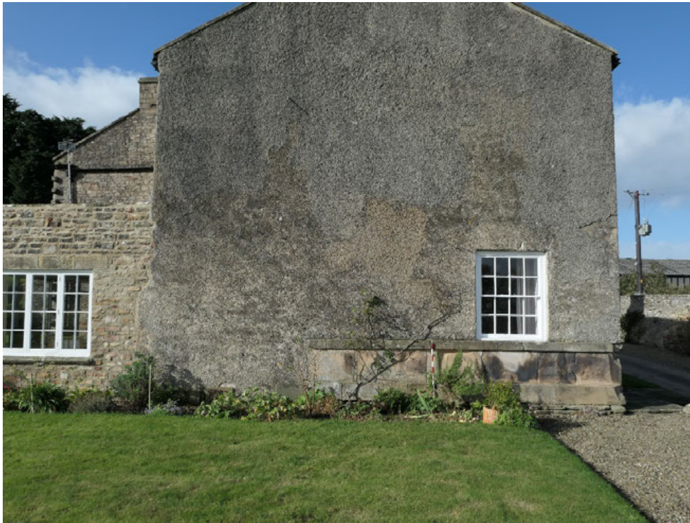
Fig. 40 Plinth course extending part way round the gable end of the farmhouse.
