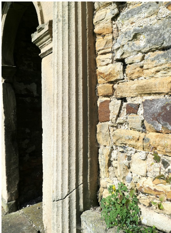
Fig. 51 Lip on the edge of a column indicating the thickness of a coat of render
