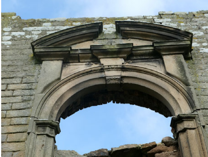
Fig. 26 Detail of the door opening on the W side of the tea house showing oak leaf decoration on the keystone of the arch
