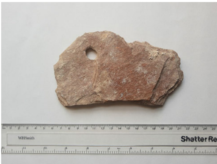
Fig. 83 Broken roofing slate?
