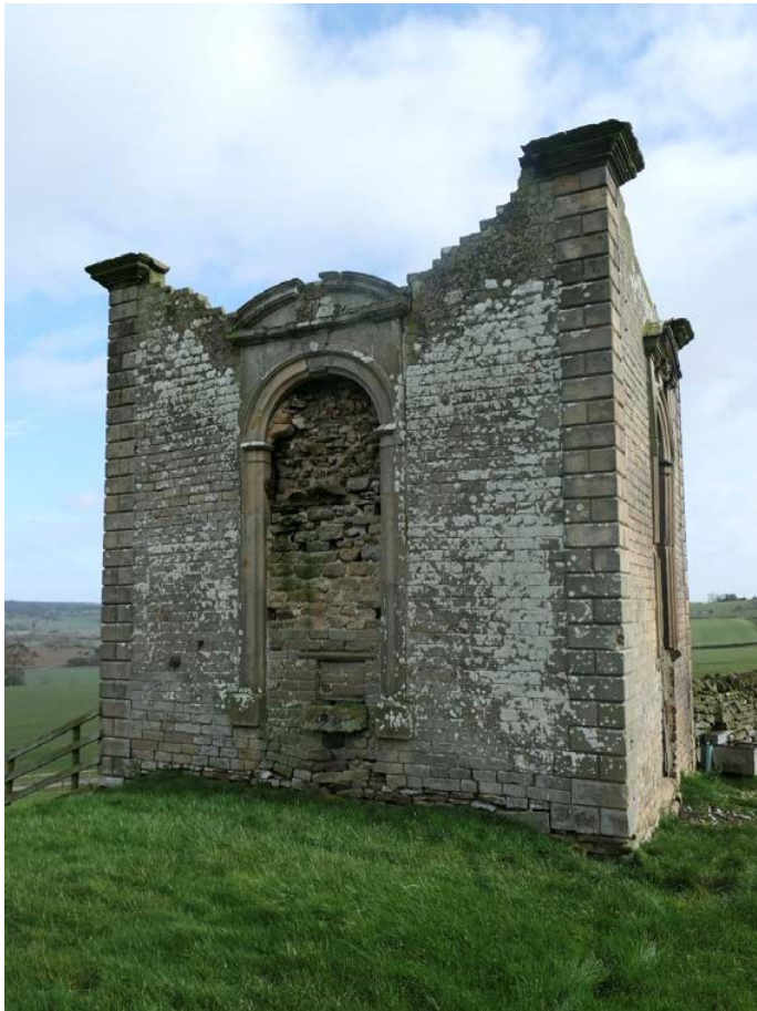
Fig. 24 The blocked doorway of the 'Bell Park' pavilion or tea-house.
