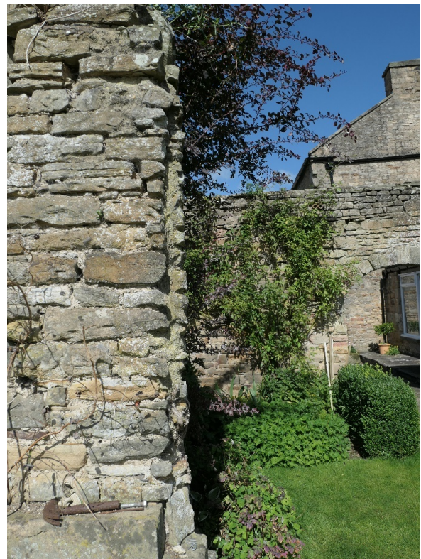
Fig. 52 The rebate in the blocking of the mullioned window designed to house the frame of a sash window. The hammer sits on the string course of the plinth believed to have been inserted by Garrett.
