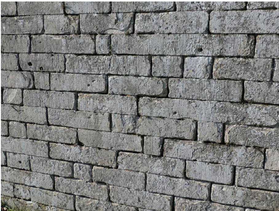
Fig. 18 Ridged tooling on the ashlar masonry of the bastioned wall.
