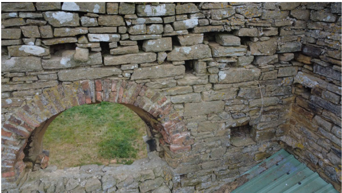
Fig. 25 Interior view of the tea house showing a window opening under a brick arch. Above it are holes for joists which supported a flat roof. (Photo by Mark Denton).
