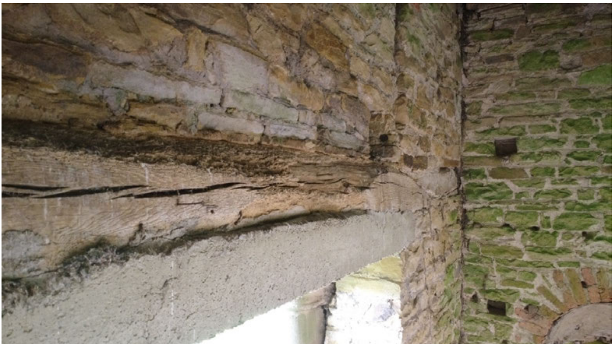
Fig. 34 A poured concrete beam was inserted in the 1970's or '80s to support the wooden beam at the front of the building. (Photo by Mark Denton).
