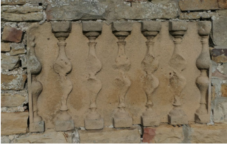
Fig. 45 Demi-balustraded panel ex situ in an outhouse wall.
