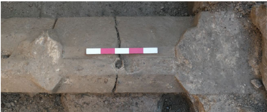
Fig. 61 Trench 1. Detail of sill showing the hole for a vertical metal stanchion fixed in place with lead which remains in situ.
