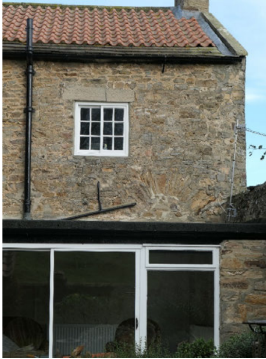
Fig. 42 The relieving arch in the rear wall of the farmhouse.
