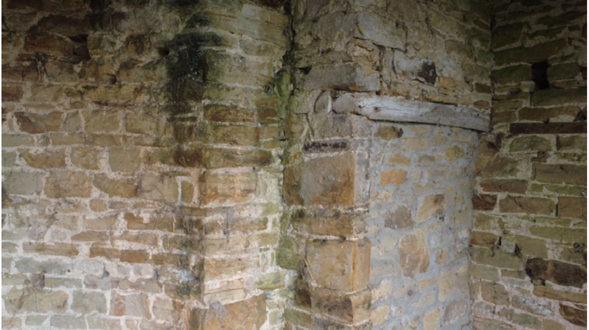
Fig. 33 The blocked doorway in the SW corner of the main chamber. (Photo by Mark Denton).
