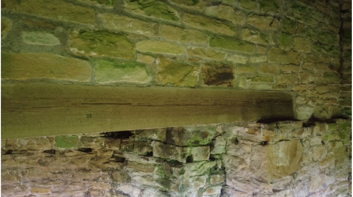
Fig. 35 A new wooden beam supports a re-built wall at the back of the main chamber and in front of the projecting apsidal element. Note the regularly spaced holes in the masonry below which may have held wooden plugs to which lathes or battens were nailed. (Photo by Mark Denton).
