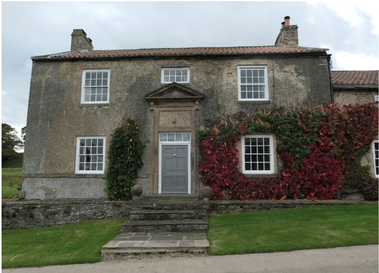
Fig. 39 The north-facing facade of the farmhouse. The string course and basal plinth extend the full width of the main façade beneath the Virginia creeper; Note the decorative stone balls which may originally have topped gate pillars belonging to the garden shown in Buck's drawing.
